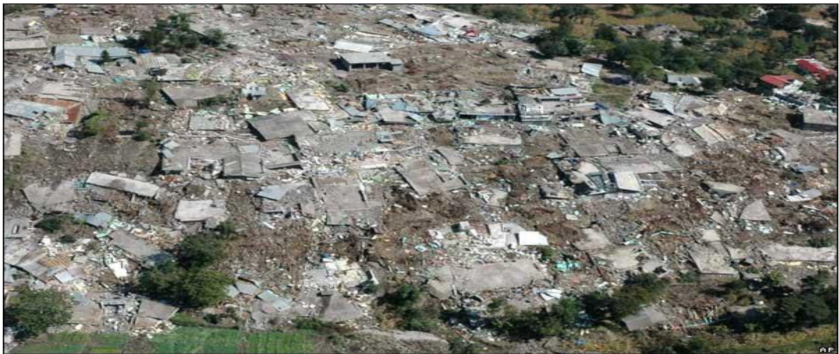
Fig. 03: The Aerial view of Destroyed Buildings & Collapsed Roofs Credit: Associated Press (AP) 2005
